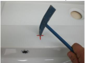
At this point strike the ceramic in the centre of the hole a number of time with a pointed hammer.
