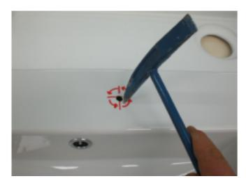
Continue opening the hole giving some gentle strikes to widen the existing hole rotating around the hole to reach a diameter of 35 mm.
