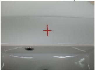
Mark the centre of the hole exactly intersecting the lines.
