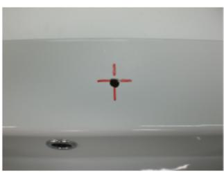
Continue to strike until a small hole is created in the upper part while in the lower part the ceramic disc has completely cleared.
