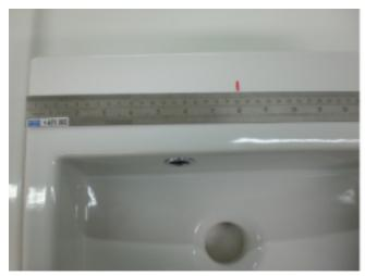
On the upper level of the tap mark the centre of the hole from the wash-hand basin side as taken from the measurement on the technical specification.
